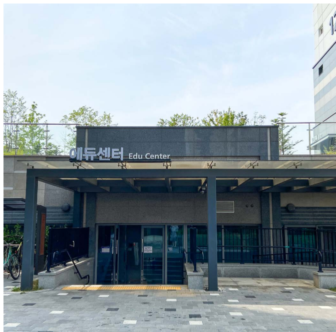
Figure 3: Yuseong Education Center exterior view.
